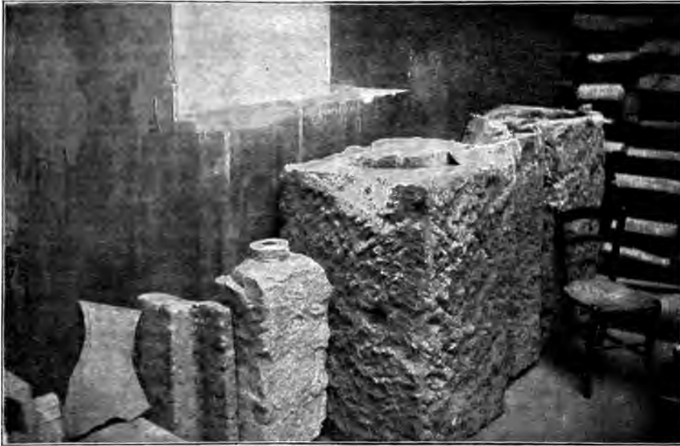
ROMAN WATER PIPE MADE OF BORED-OUT BLOCKS OF STONE. 1
